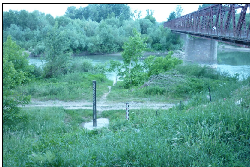
Fig. 6 The water gauge at the Tisza River Bridge in Vylok (Izhak, 2012).
