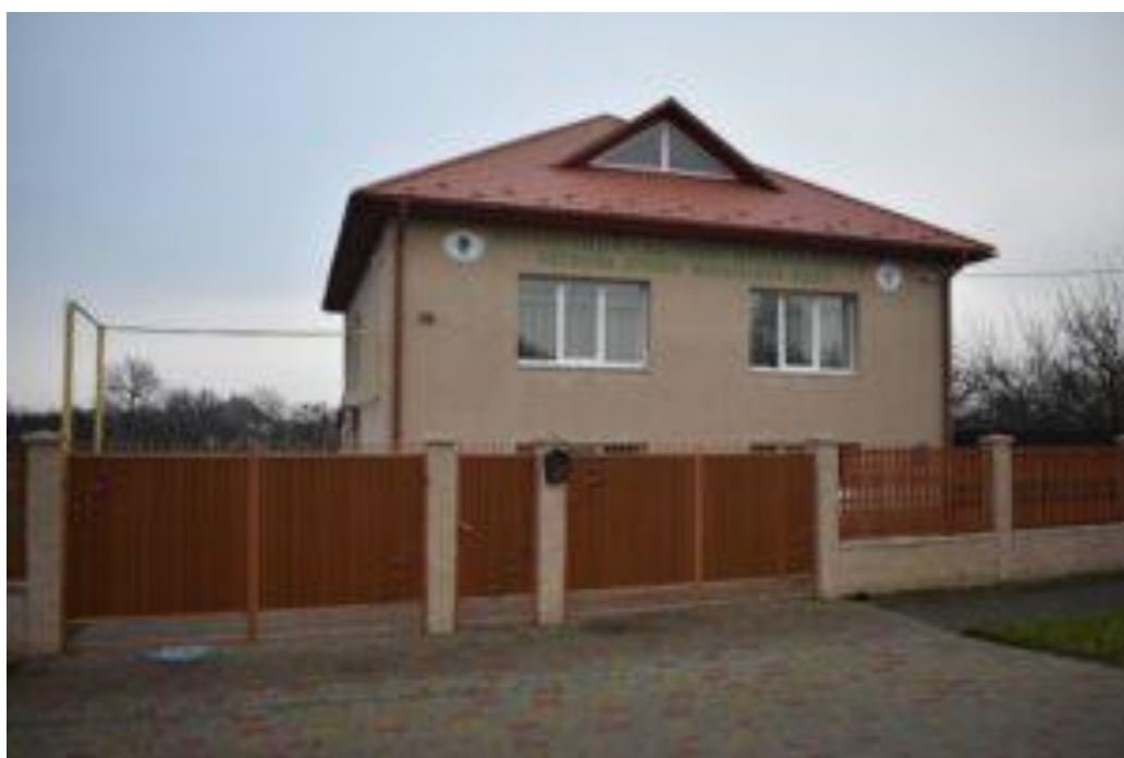
Fig. 5. The main building of the Botanical Garden
